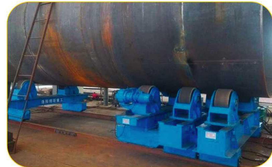
组对滚轮架应用现场 Fitting up Welding Rotators On-site
